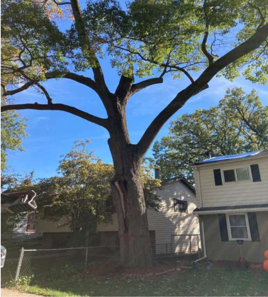
2112 Reaney Ave – Dangerous Tree
